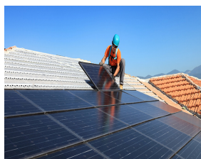
Fig-1: Installation of solar panel
