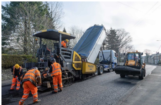
Fig-10: laying of road by using bitumen and aggregates mixing
