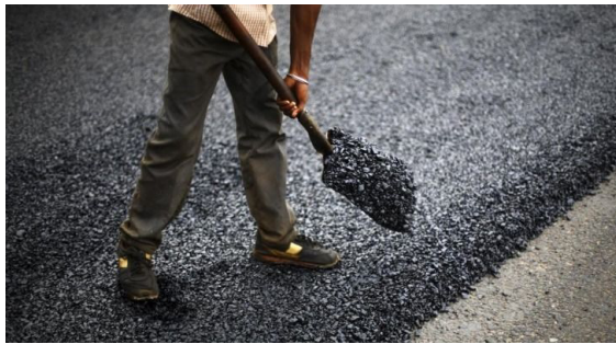
Fig-9: shredded plastic waste over the aggregate
