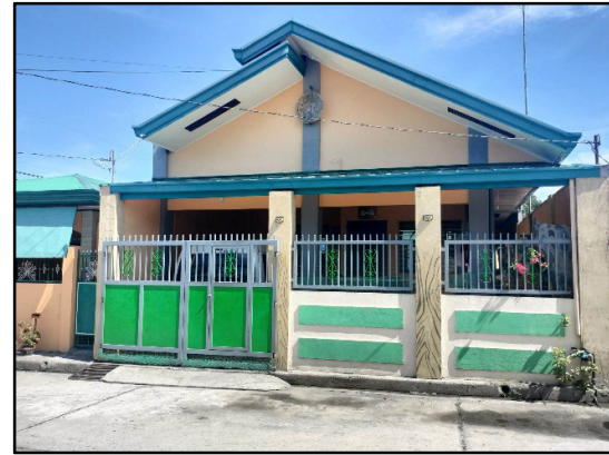
Fig. 5 Example of Good Construction of Gable Walls from Model Community, Porac, Pampanga
