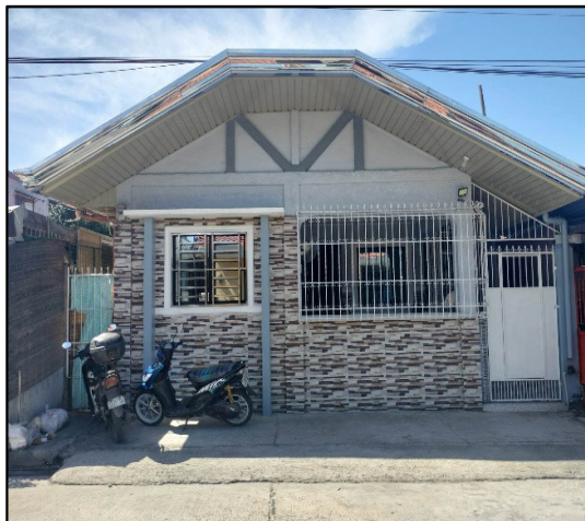
Fig. 4 Example of Good Construction of Gable Walls from Model Community, Porac, Pampanga
