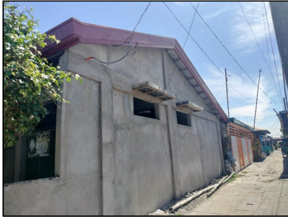
Fig. 6 Good Construction of Beams and Columns
