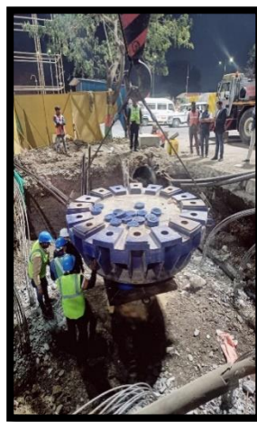
fig. 5 placing of Test Crown
