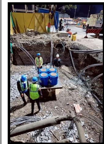
fig. 4 placing of Hydraulic Jack
