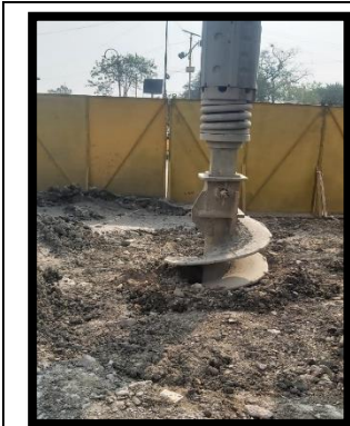
Fig. 2: boring work on the test pile
