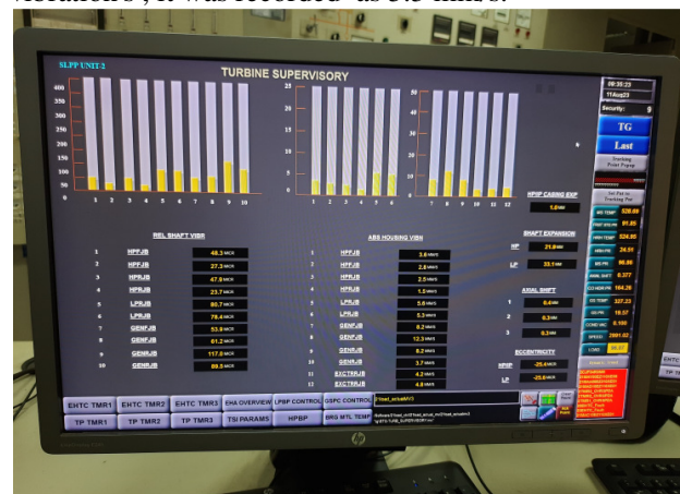
Figure 11: TG deck Vibration data after restoration
