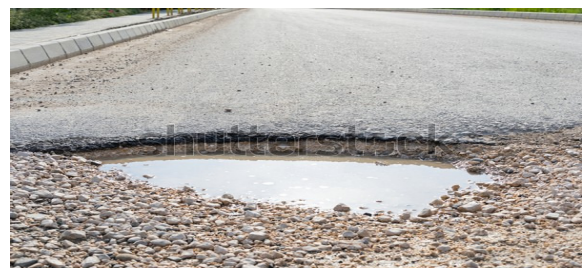
Figure 1.1 Pothole
