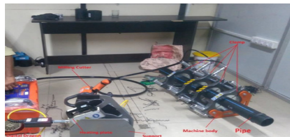
Figure 1. Butt-fusion welding set up [1]
