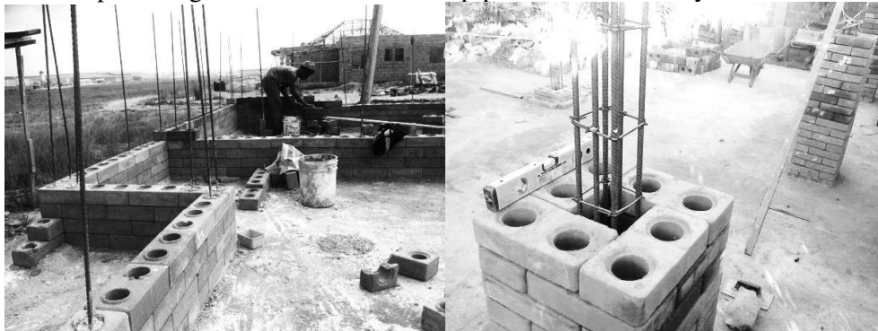
Plate 2.1: Showing reinforcement in ISSBs Source: Field study
