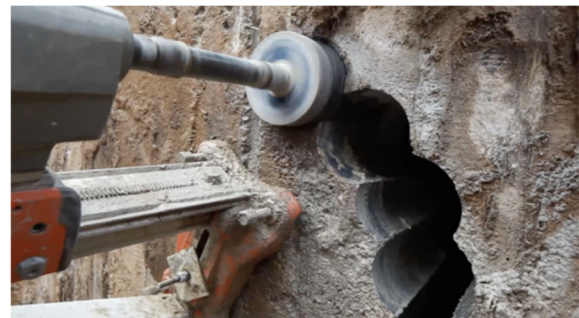
Figure7: Core Extraction Source: Internet
