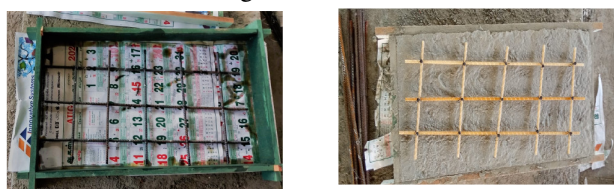
Steel reinforcement
