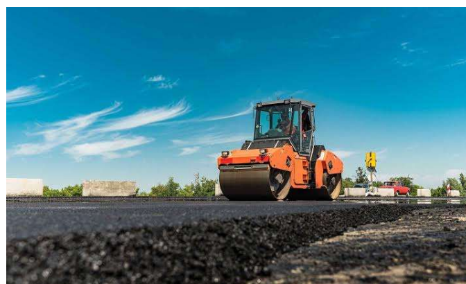
Fig. 4: Lignin-Based Asphalt Pavement in Netherlands
